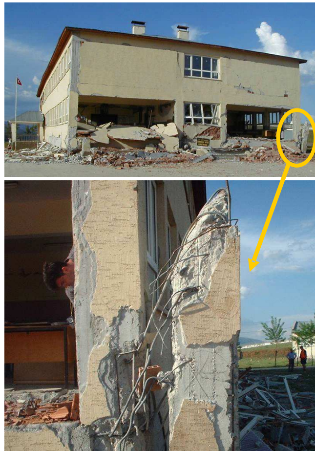
Figure 5.73 Typical confinement detail of a column in building C-13-09. The shear failure in the columns initiated the collapse of the first floor. The spacing of the transverse reinforcement is 10 cm at the top 30-cm portion of the columns. The ends of the stirrups were not anchored properly.
