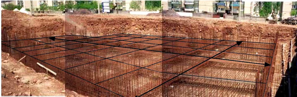
Figure 4.1 Steel in the foundation of a new hospital under construction in the north side of Bingöl. The foundation includes a grid of reinforced concrete beams with columns at the grid intersections. The alluvial deposit can be seen on the far end of the excavation; note the almost vertical cut in the granular material.
