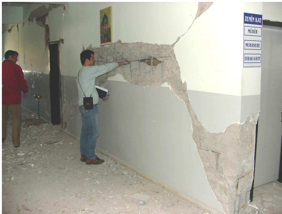
Figure 5.64 Bingöl Lisesi, school building, core concrete crushing and resulting gap in the shear wall
