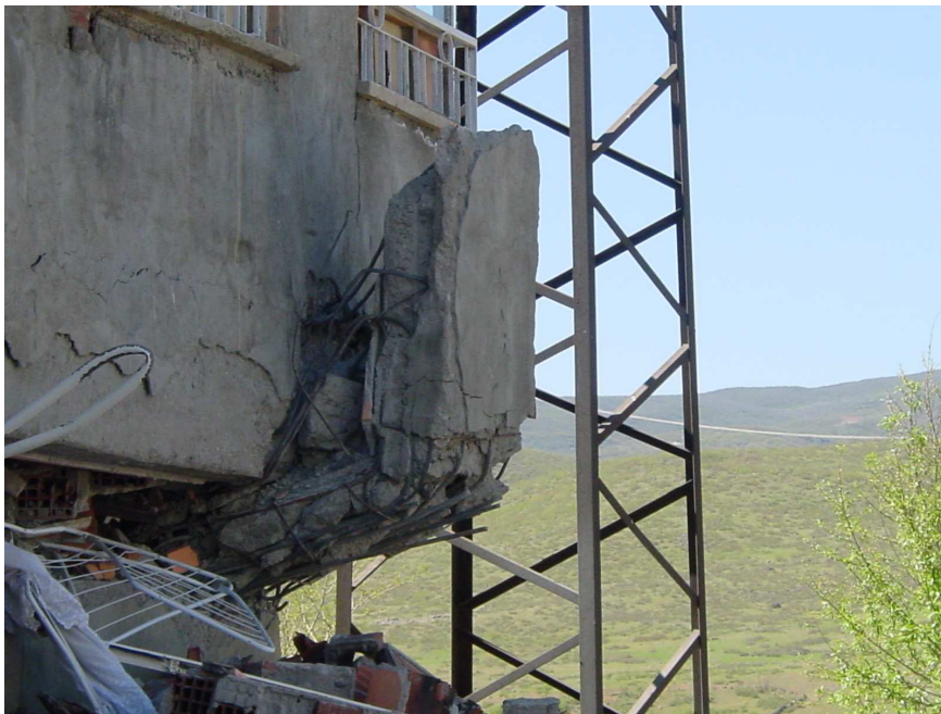
Figure 5.19 Insufficiently confined column of a collapsed building
