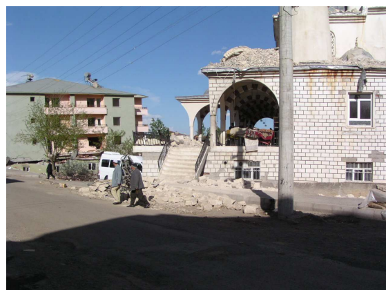
Figure 5.85 View of Yenimahalle mosque with the private residential building that lost its 2nd story.
