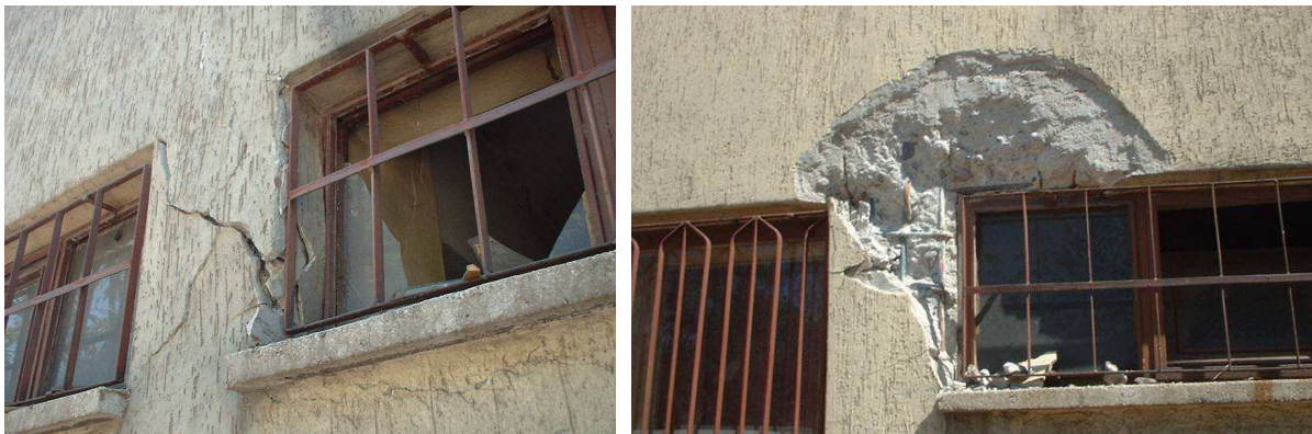
Figure 5.71 Shear failure of captive columns created by the small windows of the furnace room in building C-14-03.
