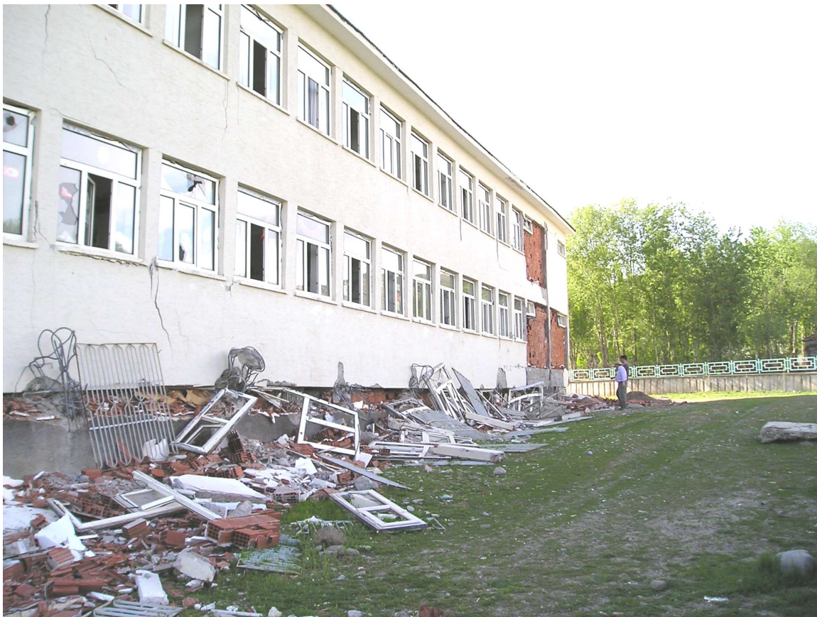
Figure 4.3 School with collapsed first floor in NE Bingöl. Note that first floor is missing. Windows were in the first floor. Cracks in soil near foundation were at far end of building.
