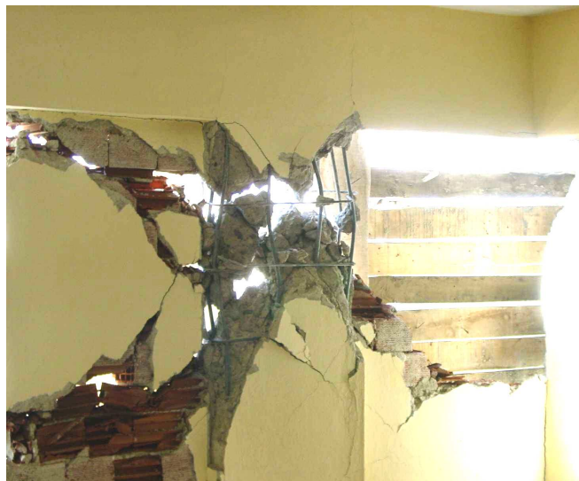
Figure 5.32 Brittle failure of the column of building shown in Figure 5.30. Buckling of bars due to insufficient lateral confinement and crushing of core concrete.
