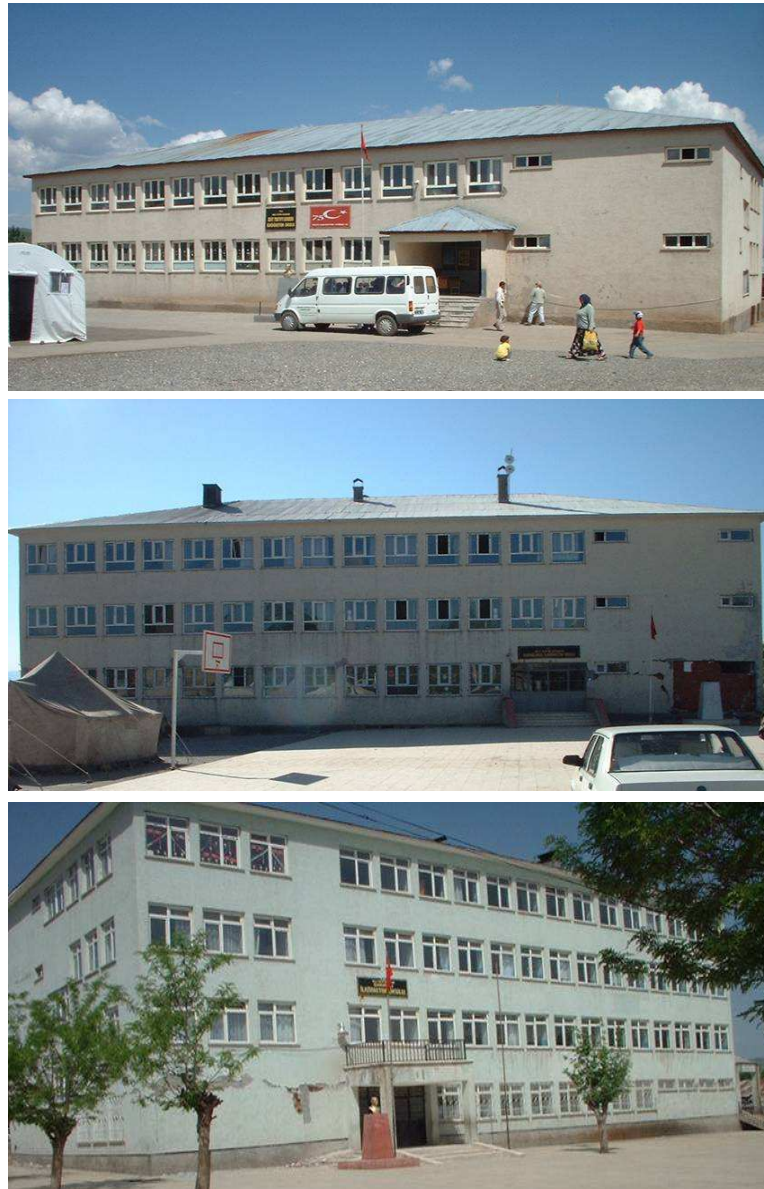
Figure 5.69 School buildings with typical floor plan. Column dimensions are the same regardless of the number of floors.
