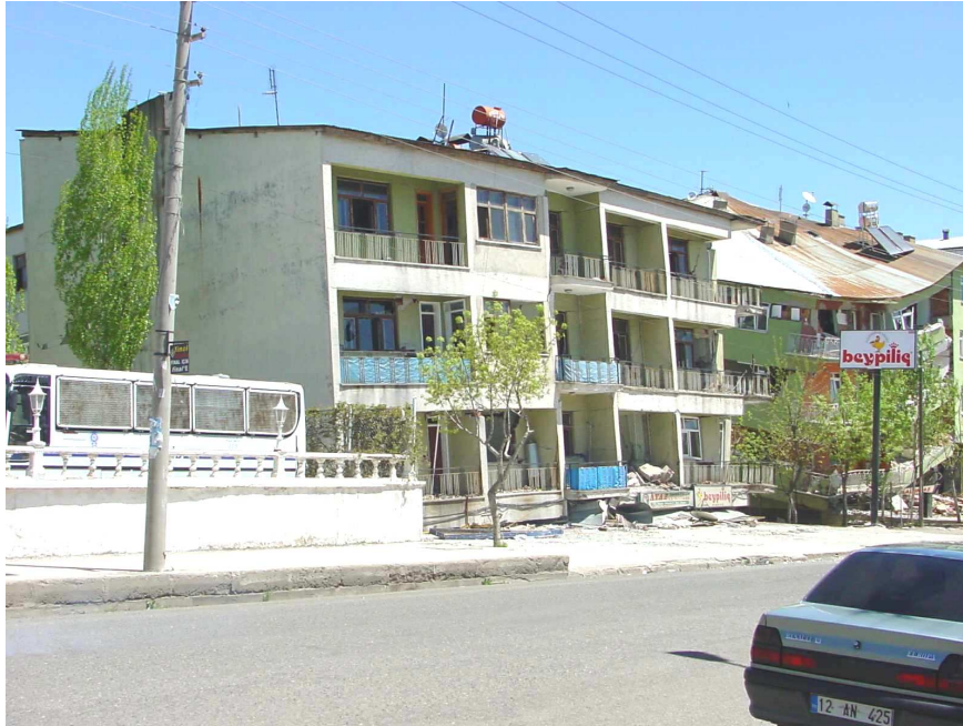
Figure 5.14 First story collapse of a four-story building
