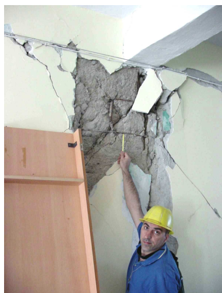
Figure 5.11 Diagonal tension crack at the upper end of the ground floor column
