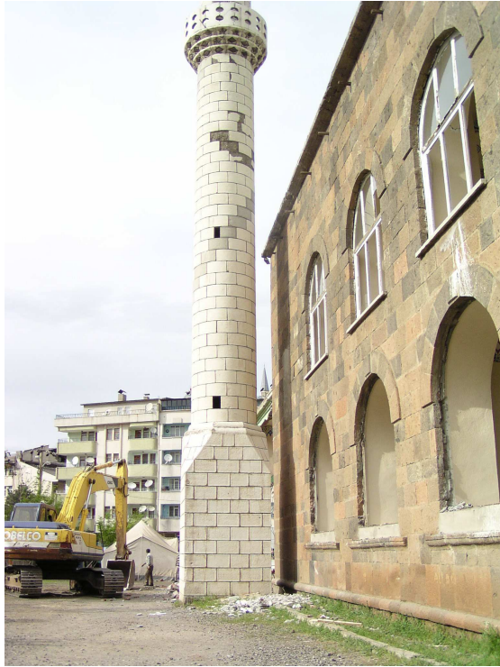
Figure 5.86 Yeni/Hacılar mosque with spalling in its minaret. The structure is being demolished.
