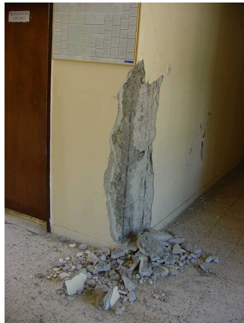
Figure 5.61 TEDAŞ Bingöl branch, inadequate confinement at column ends
