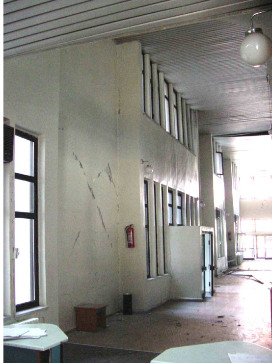
Figure 5.58 Diagonal cracks on partition walls (Ziraat Bankası, State Agricultural Bank)
