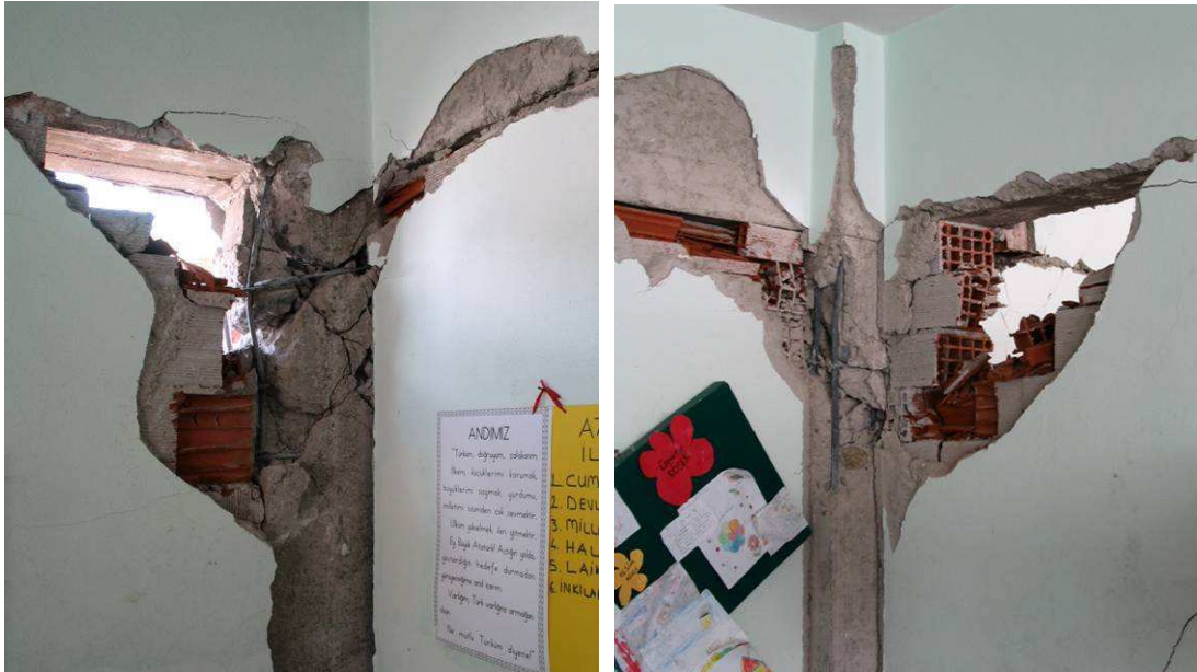
Figure 5.72 Shear failure of captive columns as a result of crushing of upper corner of masonry walls in building C-14-01.
