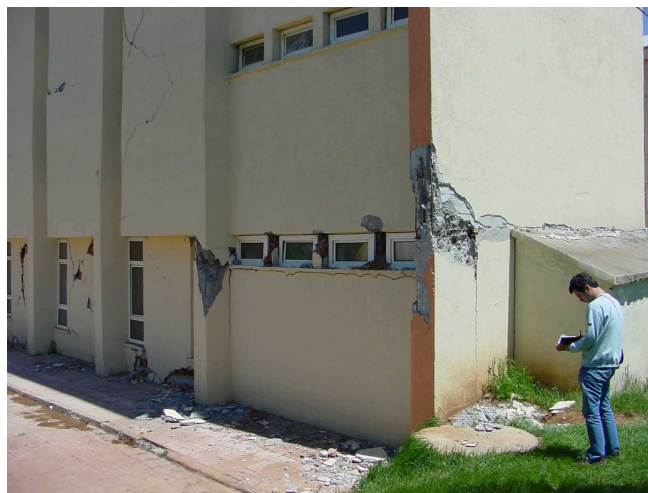
Figure 5.62 TEDAŞ Bingöl branch, damage in column end zone due to short column effect
