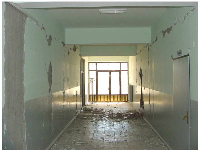
Figure 5.66 Bingöl Lisesi, school building, diagonal cracks in the infill masonry walls
