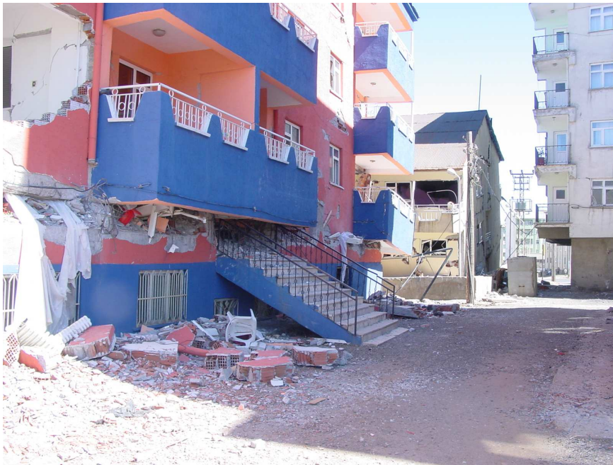
Figure 5.17 Loss of soft story in reinforced concrete frame building
