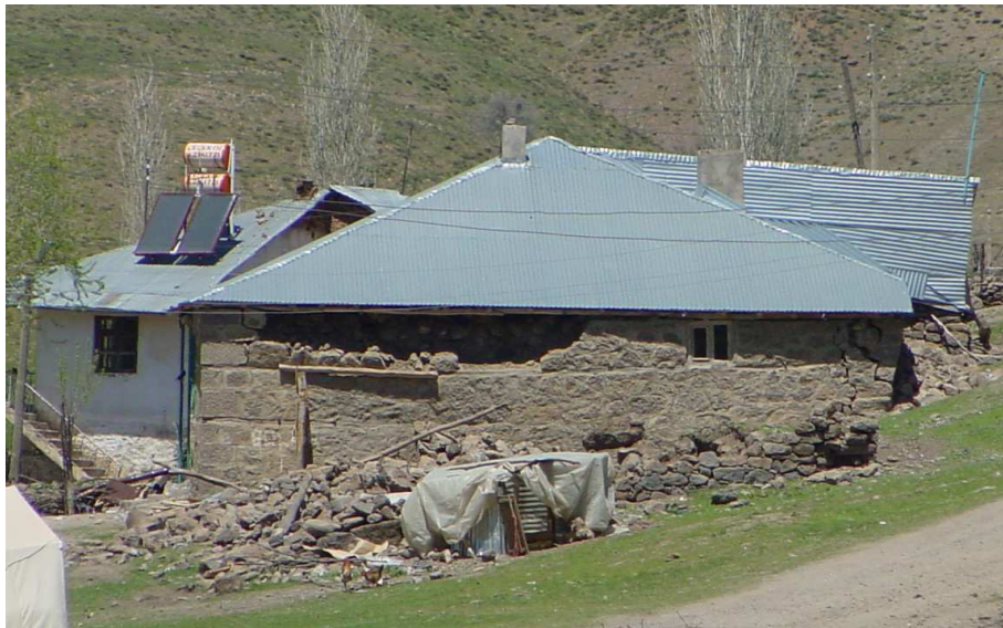
Figure 5.93 Partial collapse of hybrid masonry walls (bricks and horizontal wooden layers)
