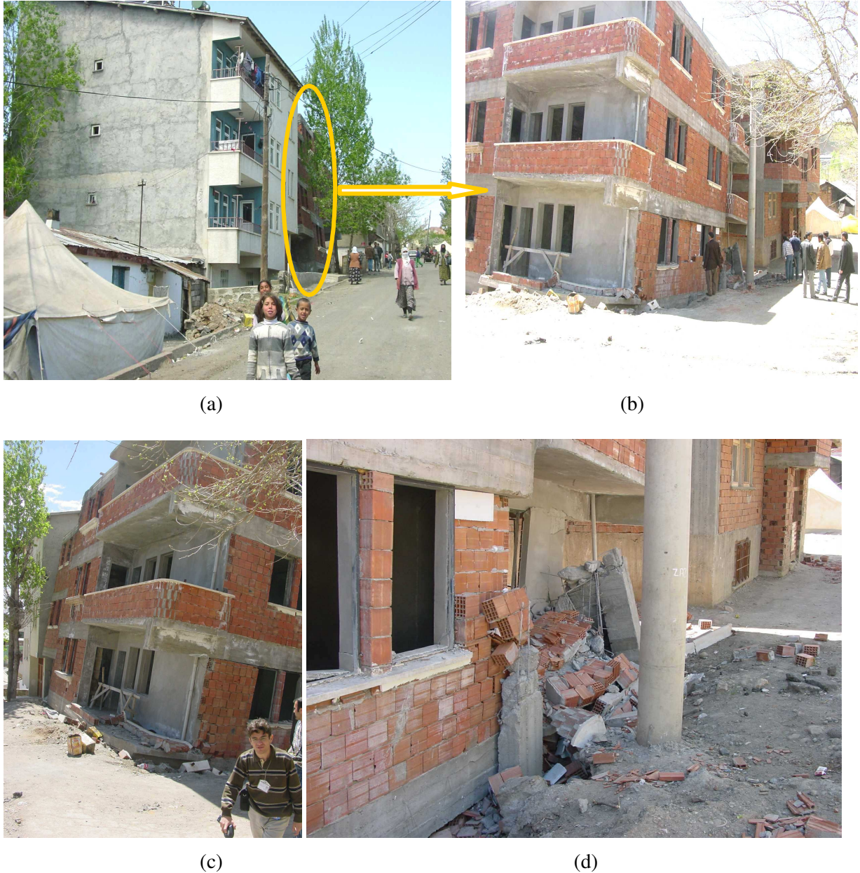
Figure 5.22 a) Lightly damaged four story RC building constructed in 1996; b, c) Complete damage to four story RC building constructed in 2003; d) Column offsetting at collapsed floor due to improper connection.
