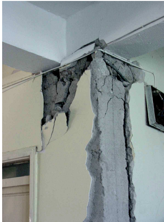
Figure 5.13 Column damage and condition of beams
