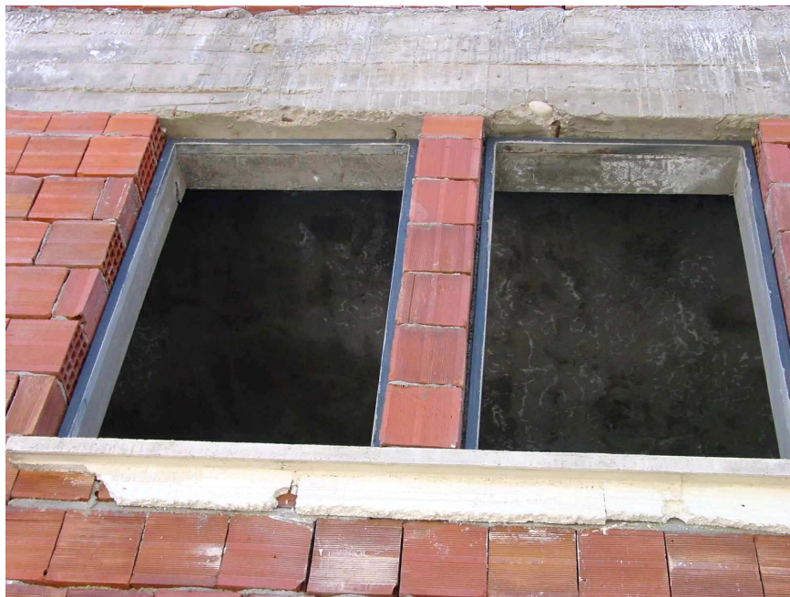
Figure 5.28 Window framing detail. Steel frame is welded to the rebar of the beam.
