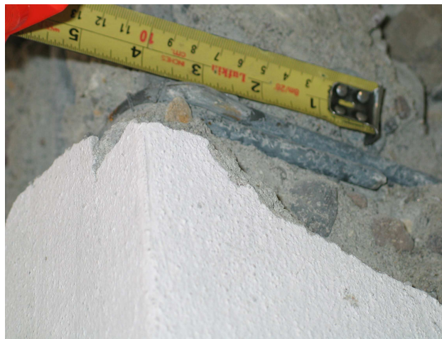
Figure 5.47 Typical detail for anchorage of stirrups
