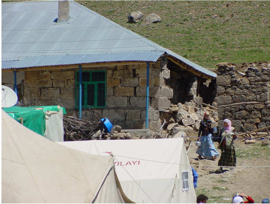
Figure 5.95 Stone-masonry type wall collapse
