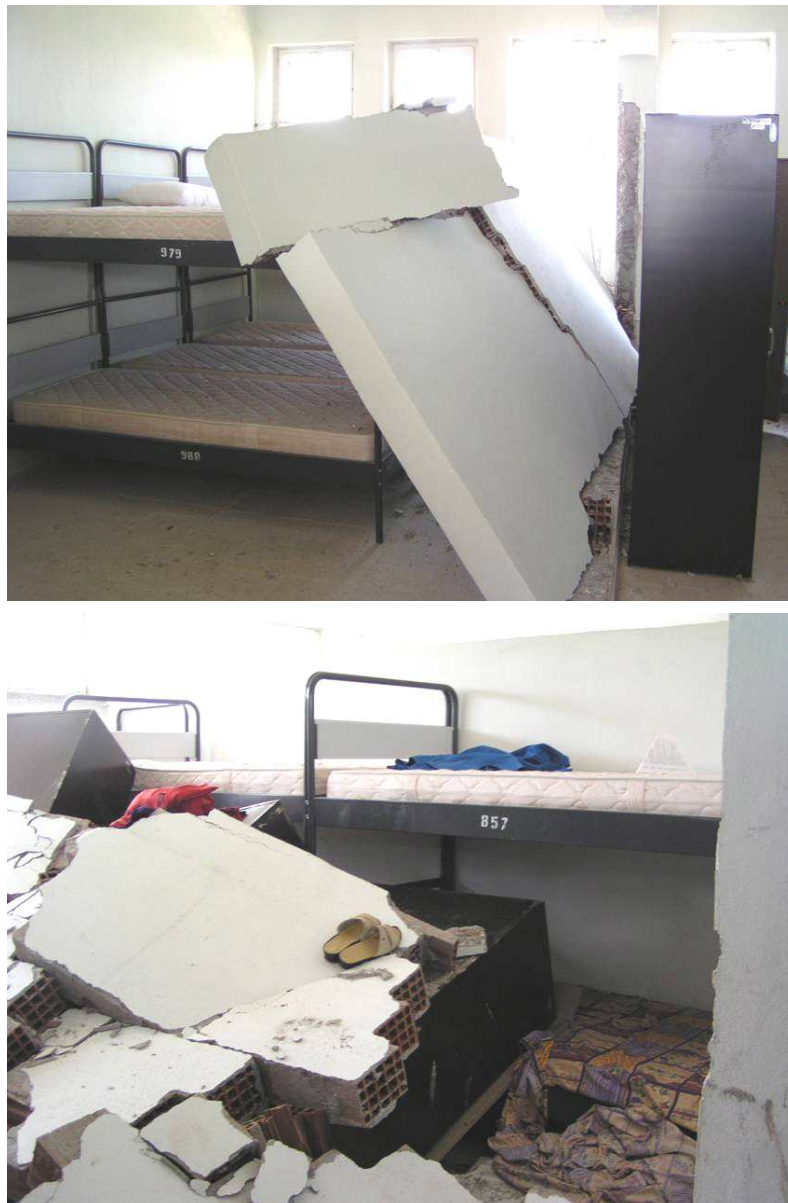
Figure 5.79 Collapse of the free standing masonry walls onto the beds in the dormitory buildings.
