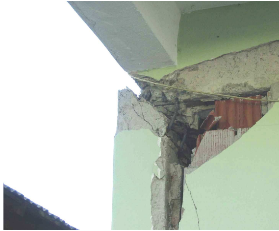
Figure 5.34 A corner column on the ground floor of a four-story building. Separation of the column due to improper detailing.
