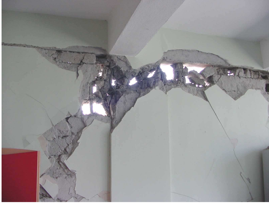
Figure 5.12 A clear column-end failure and masonry wall damage
