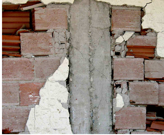
Figure 5.33 An inclined shear crack of a moderately damaged column.
