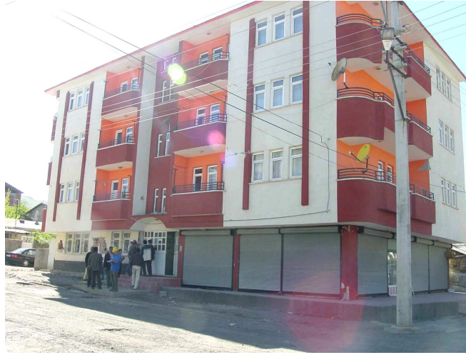
Figure 5.30 Four story residential building. The look from outside is quite different and misleading for a heavily damaged building.
