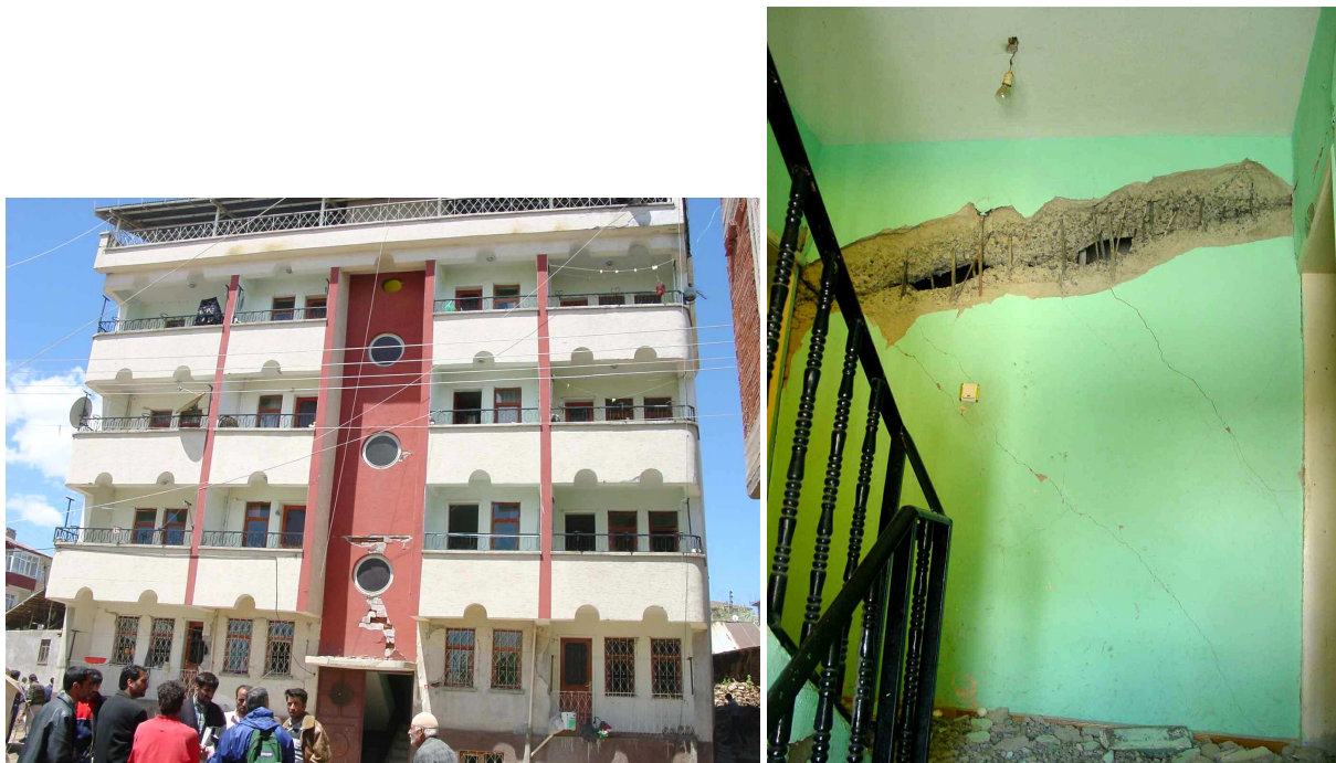
Figure 5.26 Heavily damaged 4 -story building (plus penthouse) and the damage experienced by its shear wall
