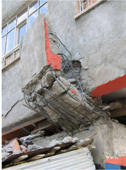
Figure 5.46 Typical location of column splice
