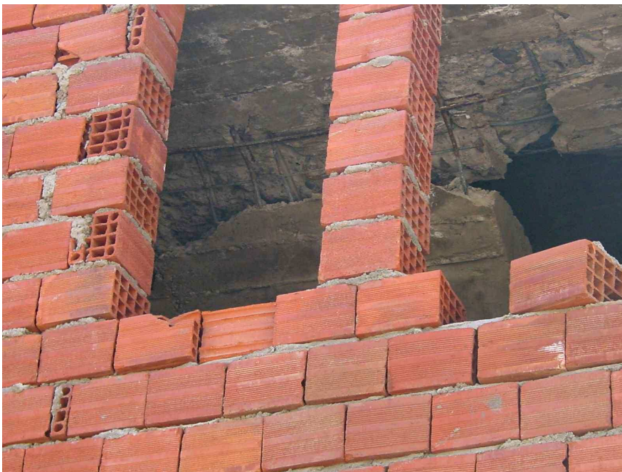
Figure 5.8 Typical hollow clay tile used in infill walls
