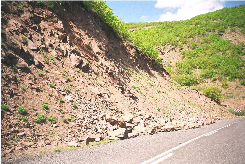
Figure 4.22 Rock falls near Gökçekanat (Point 5 in Figure 4.13) (N 380 58.6', E 400 17.05'). Joint has a dip angle of 50 degrees to the North; strike is from east to west
