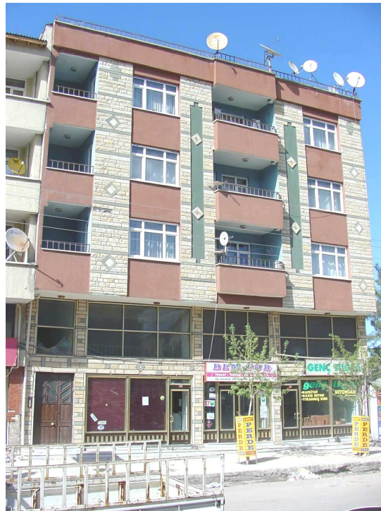
Figure 5.15 Lightly damaged five-story reinforced concrete frame building
