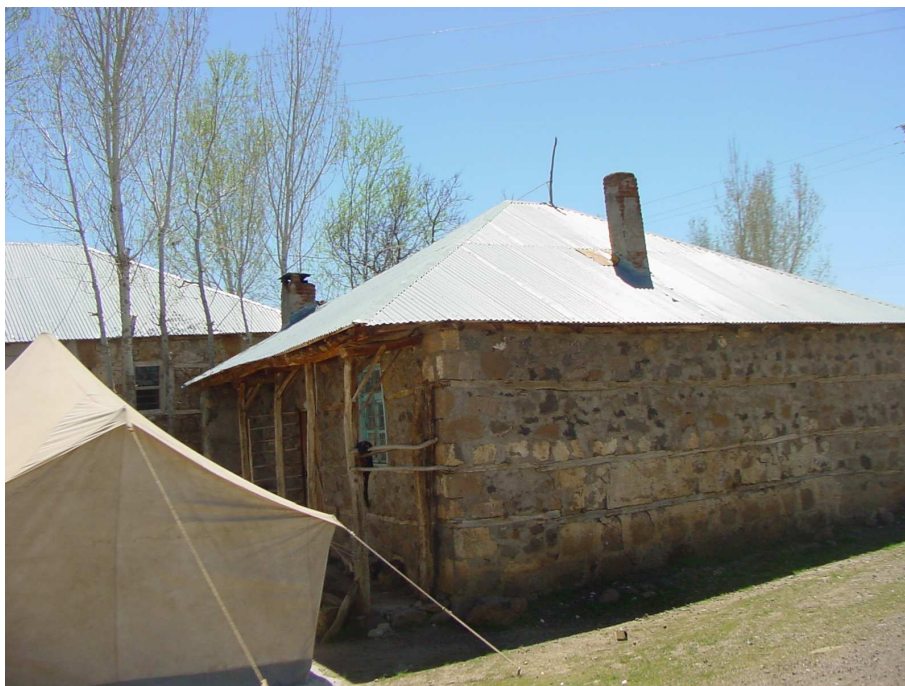
Figure 5.92 Hybrid masonry construction in rural areas (bricks and collar beams in the form of all-round horizontal wooden layers)
