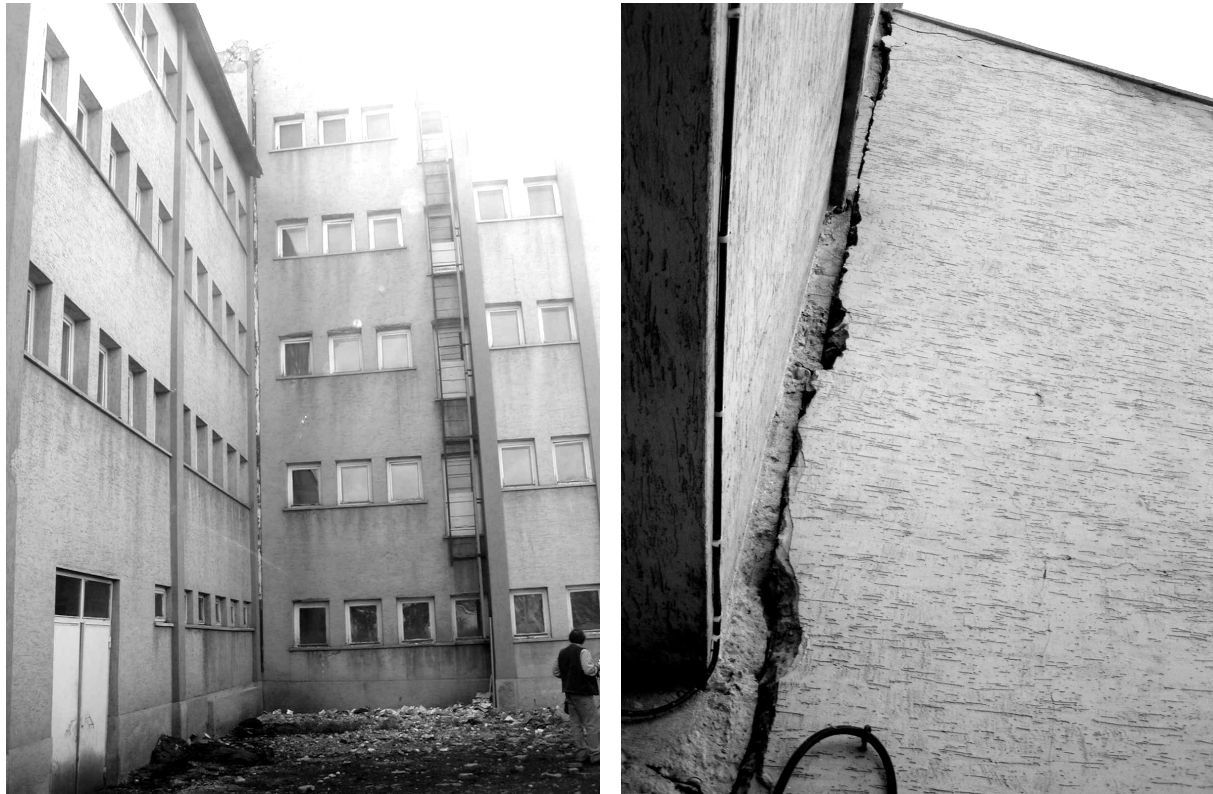
Figure 2.11 Evidence of pounding between the mid-rise office buildings of the Bingöl Public Works and Settlement branch complex. The photograph on the left is taken from the enclosed garden surrounded by the office buildings and the 1-story auxiliary structure where the strong ground motion instrument was located. The distance between the office buildings and the auxiliary structure is approximately 15m. The image on the right shows that the effect of pounding grows with height. The pounding is significant in the NS direction.
