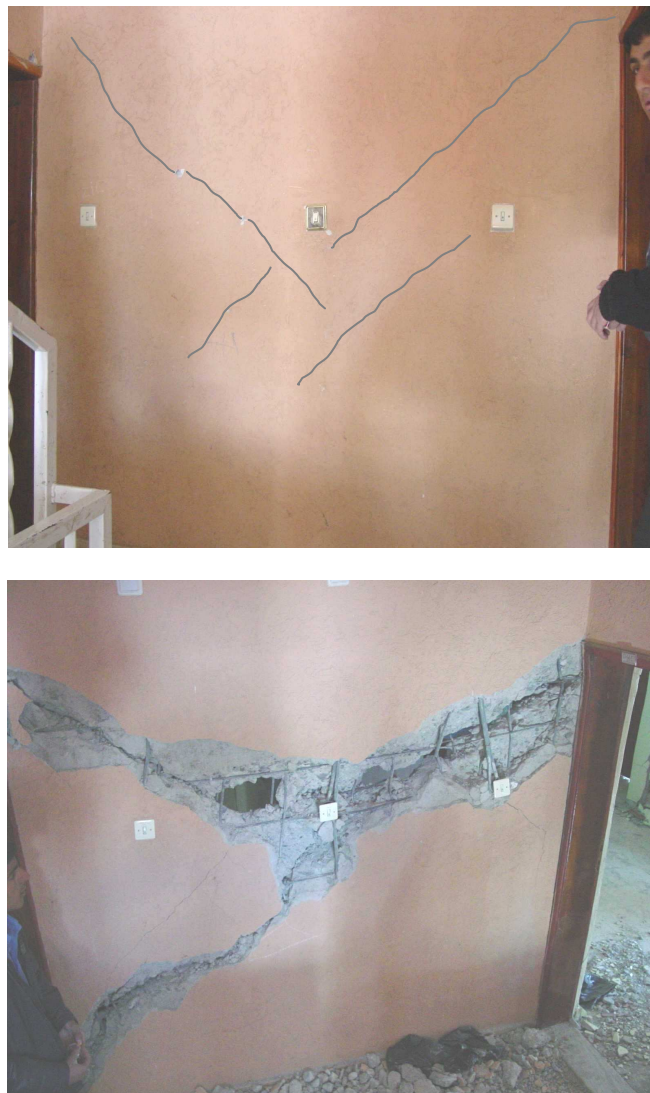
Figure 5.23 Heavily damaged reinforced concrete frame with shear wall type construction
