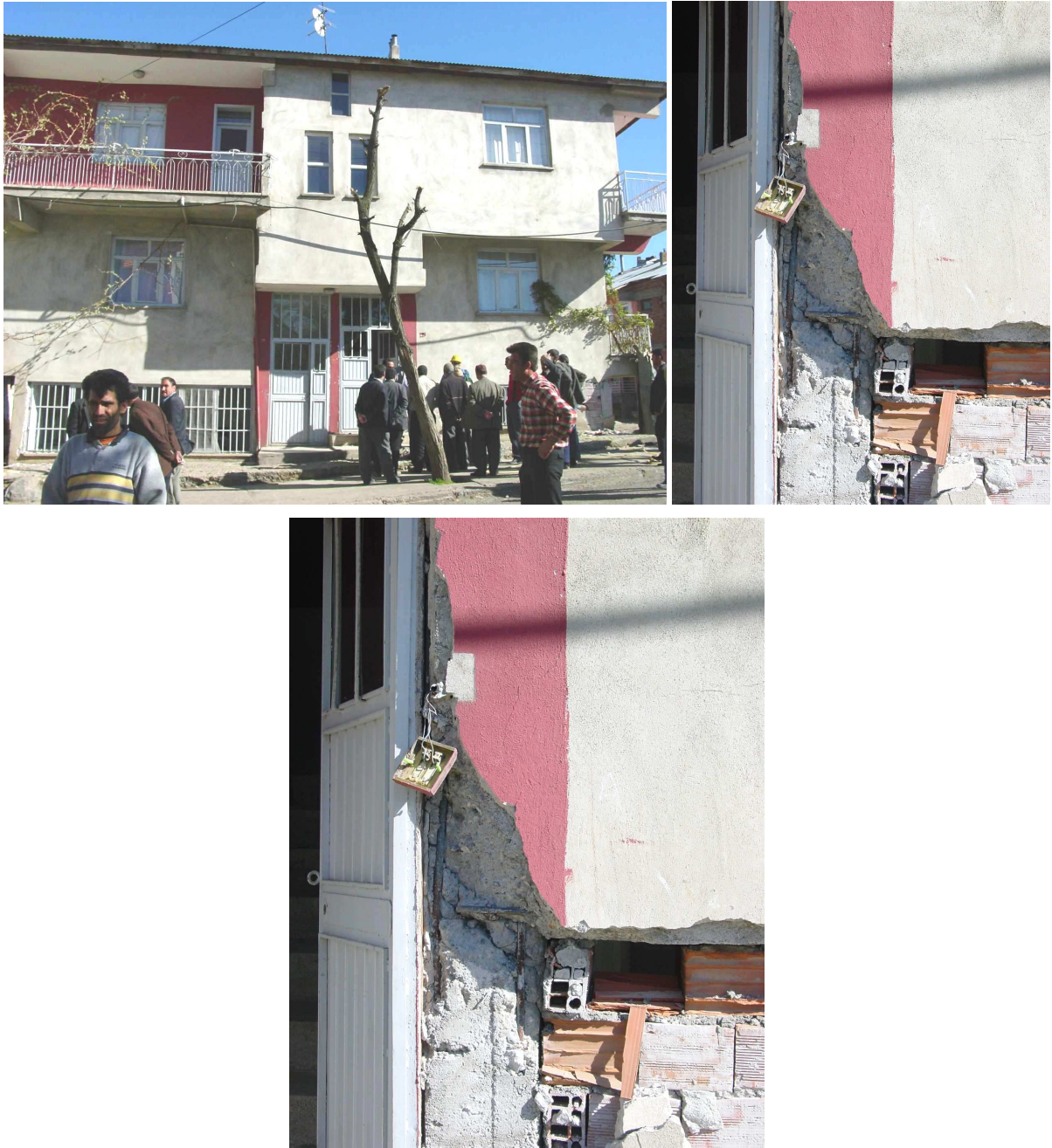
Figure 5.29 Short column damage of a two-story reinforced concrete frame building in Yeşilyurt.
