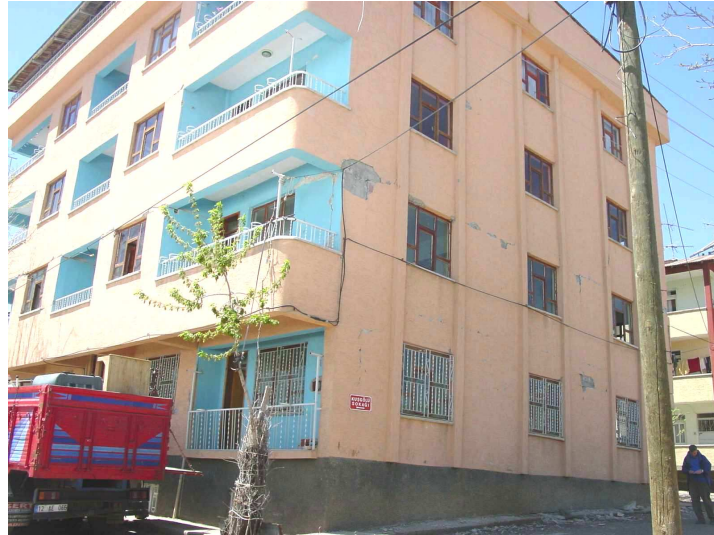
Figure 5.23 Heavily damaged reinforced concrete frame with shear wall type construction
