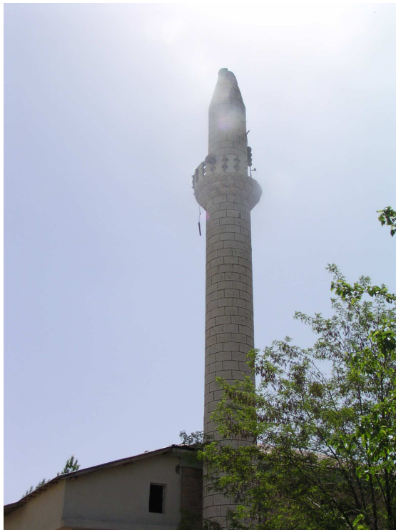
Figure 5.87 Mosque next to Sarayıçi primary school. Minaret lost its tip and part of its rail guard.
