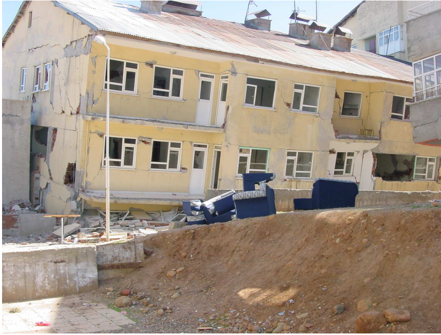
Figure 5.18 Collapse of ground floor
