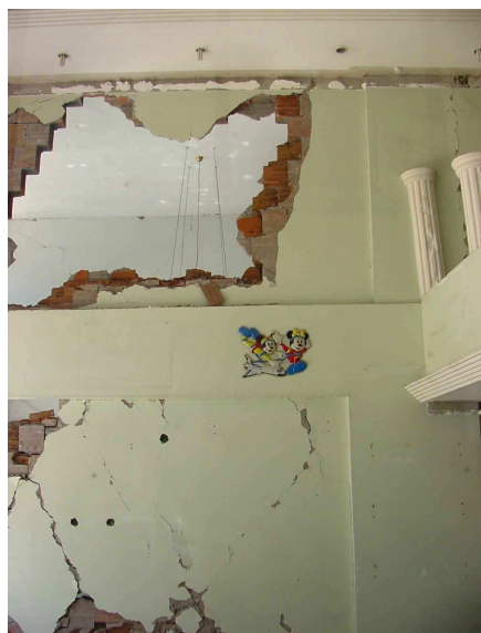
Figure 5.9 Severe infill wall damage
