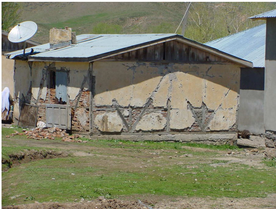
Figure 5.91 Hybrid masonry construction in rural areas (bricks and diagonal wooden struts)
