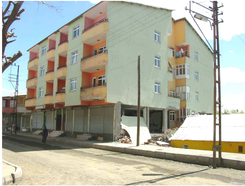
Figure 5.20 A heavily damaged four-story building in Yenimahalle
