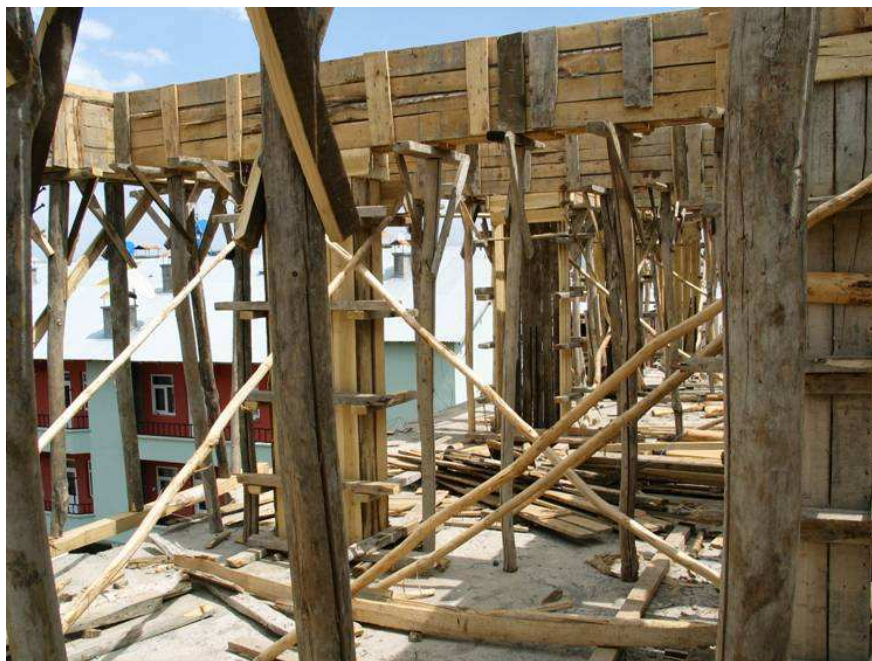
Figure 5.43 Beam and column formwork in building under construction
