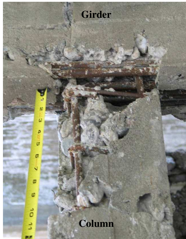
Figure 5.42 Beam-column joint in building under construction
