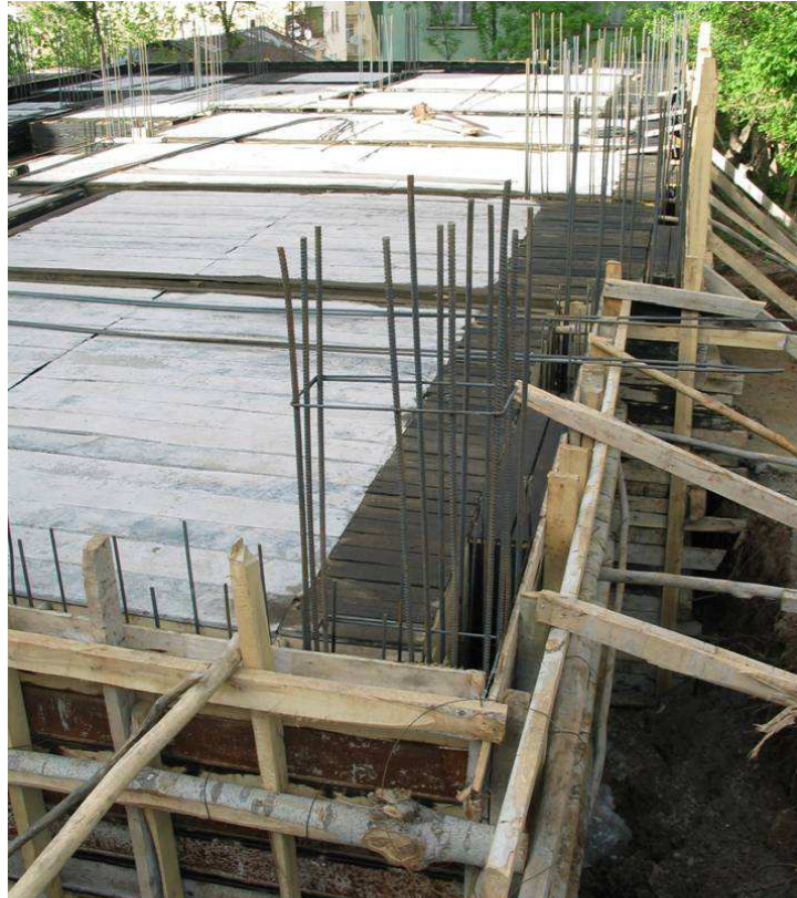
Figure 5.44 Slab formwork in building under construction
