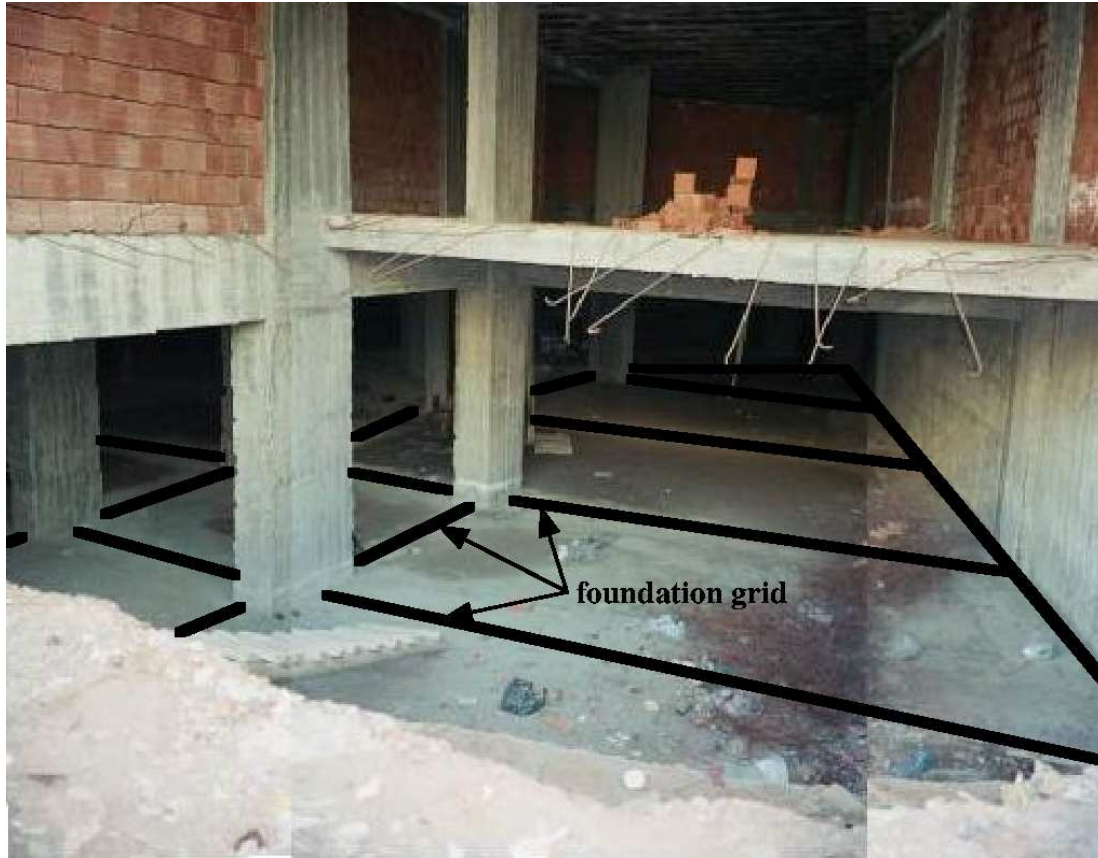
Figure 4.2 The basement of a building under construction in the south part of Bingöl. The lines mark the grid of foundation beams. The space between the beams is generally filled with gravel (from river deposits), sometimes on top of a small layer of concrete placed at the bottom of the excavation.
