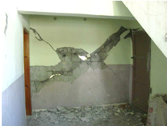
Figure 5.31 Failure of the shear wall due to inferior material quality and detailing.
