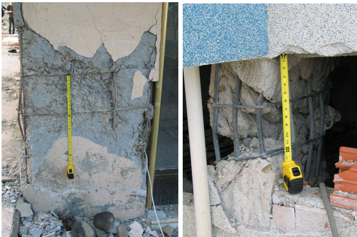
Figure 5.45 Typical column details in plastic hinge regions
