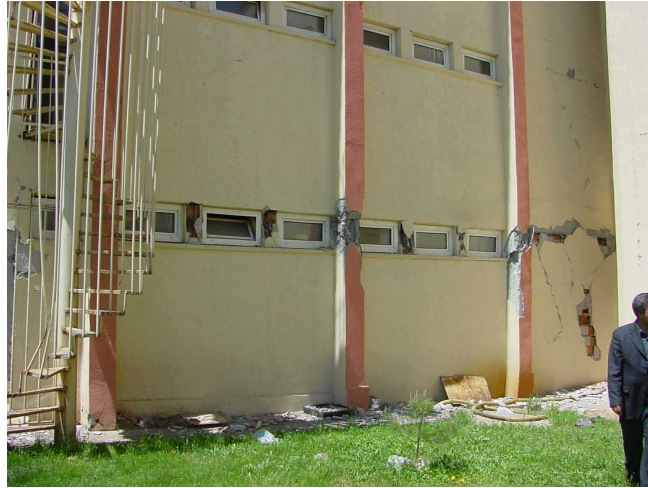
Figure 5.60 TEDAŞ Bingöl branch, short column effect
