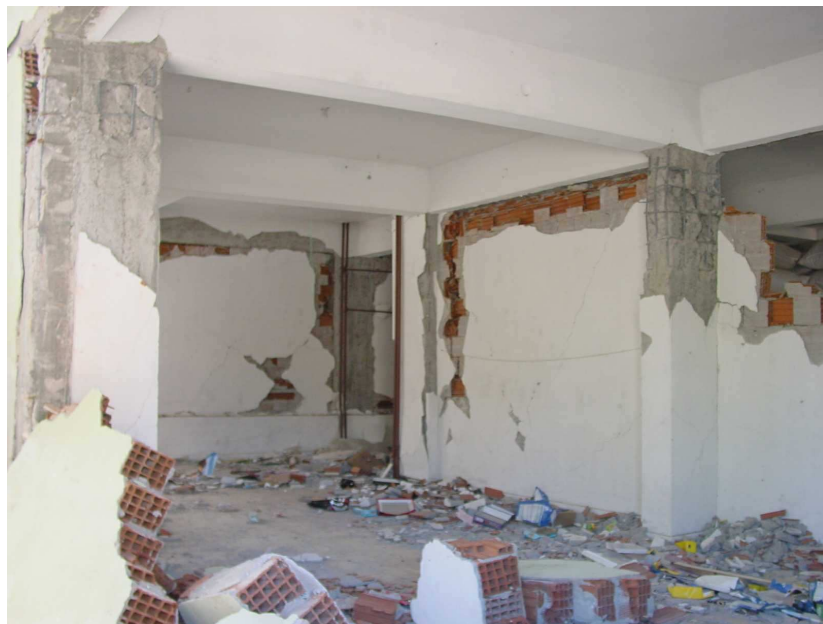
Figure 5.21 Spalling and crushing of concrete due to high axial loads
